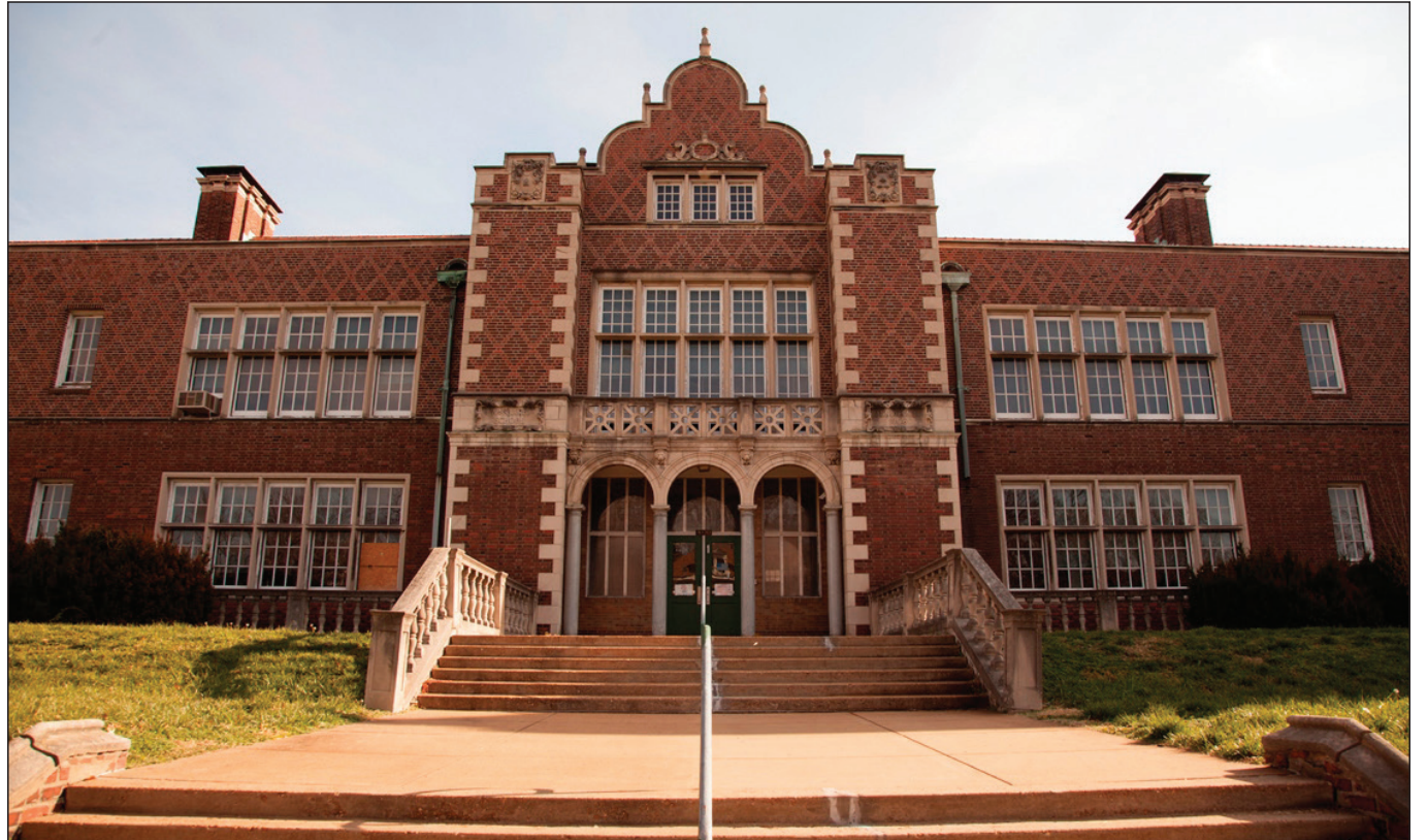
The Clark school building is located at 1020 N. Union Blvd. This historic school is just north of Delmar Boulevard with commercial areas nearby. The W.B. Ittner-designed school was named for explorer William Clark.
